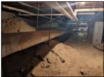
VIEW OF ACM PIPE INSULATION
