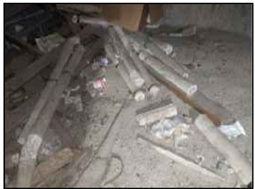
VIEW OF ACM DEBRIS ON CRAWLSPACE FLOOR
