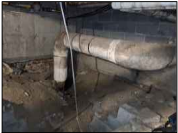
VIEW OF STEAM LINE & ACM INSULATION
