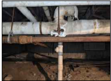
VIEW OF ACM PIPE INSULATION
