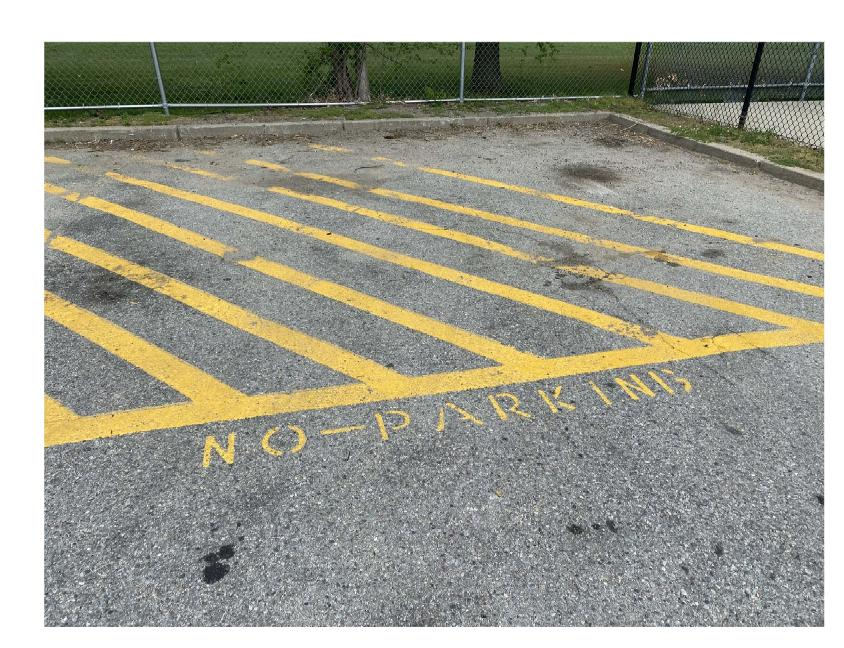
"NO PARKING" PAVEMENT MARKINGS SHALL BE YELLOW WATERBORNE PAINT 9 INCHES HIGH BY 4.5 FEET WIDE.
